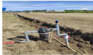
Gambar 11. Pemasangan filter SHC
